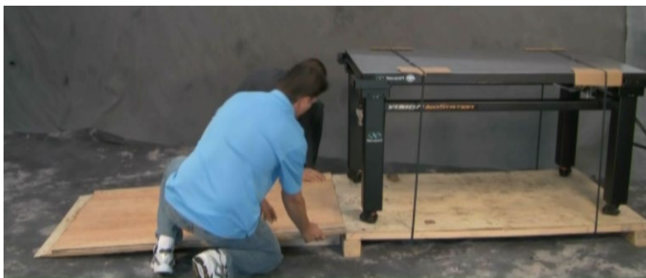
Figure 4: Vision IsoStation "roll off" ramp installation.
